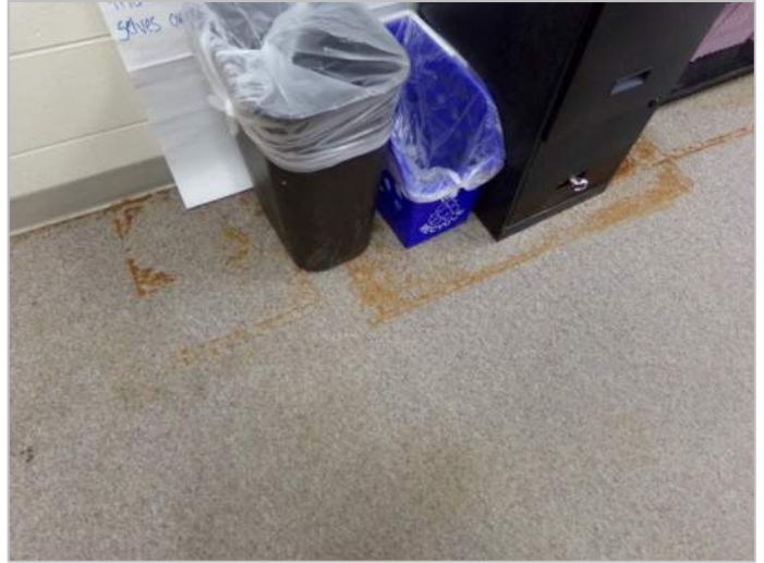
Photograph 10. View of typical water staining on carpeting. Carpet was dry at the time of our assessment.
