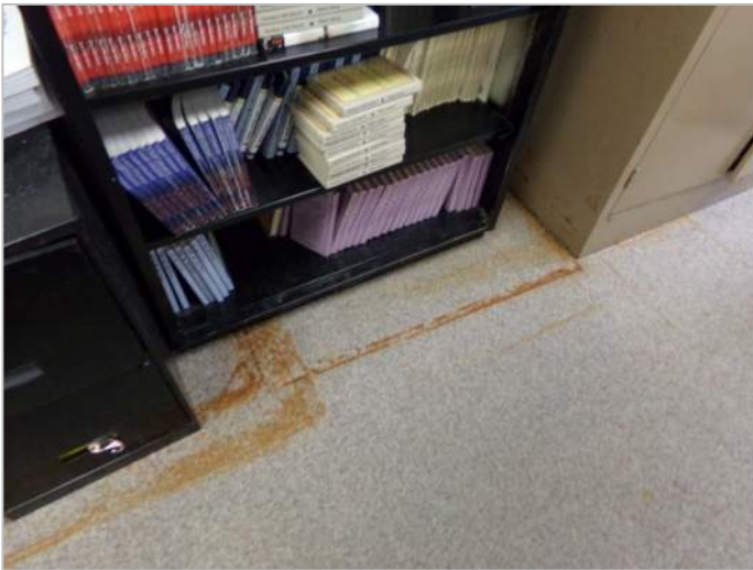
Photograph 11. View of typical water staining on carpeting. Carpet was dry at the time of our assessment.
